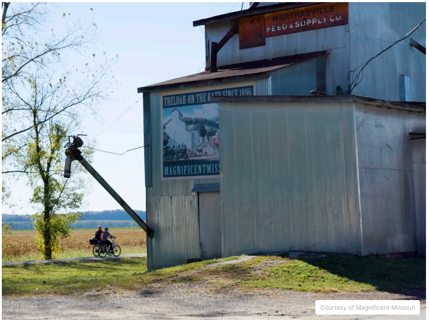
Treloar Grain Elevator along the Katy Trail
